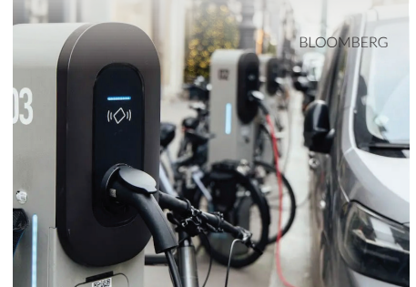
Charging stations for electric vehicles in Paris, France
